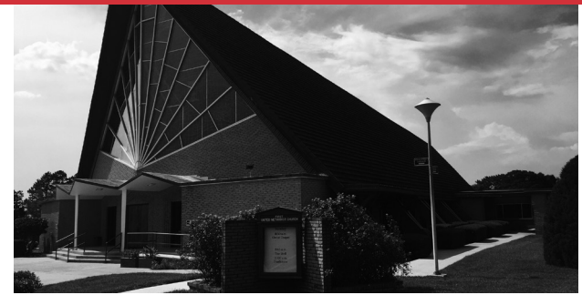
Crestview UMC worked with the Development Fund by receiving a loan to replace their air-conditioning unit.
